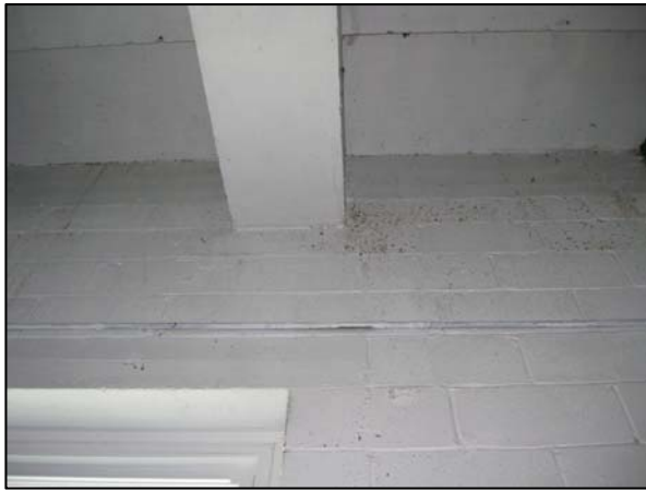
The end wall indicating the concrete beam supporting the bleachers
